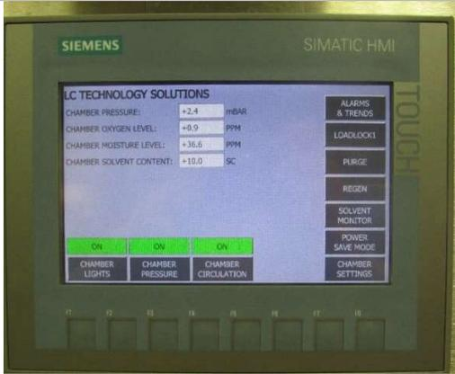
To view the Chamber Pressure, Moisture, and Oxygen Trend, press the Alarms & Trends button.
