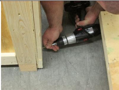
3. Use a cordless drill with a Phillips head driver bit to remove screws.
